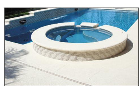
This patio pool deck has been resurfaced with Spraydeck® which is applied to both the coping and deck over existing concrete and coping
