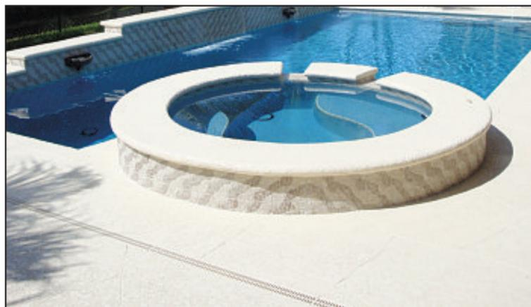
This patio pool deck has been resurfaced with Spraydeck® which is applied to both the coping and deck over existing concrete and coping bricks.
